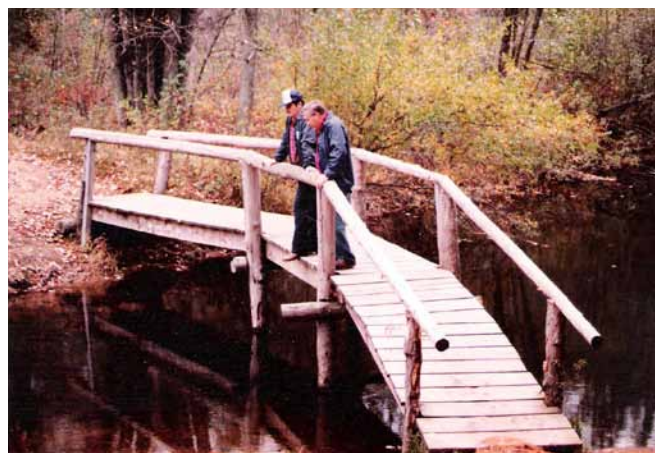
Chuck Nagel and Tony Krier, circa 1977, reflecting on the bridge over Cleveland Creek. Tony had recently completed its construction.
