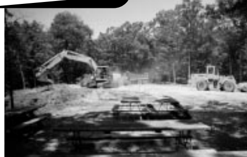
Cleaning Up the Carlen Debris
